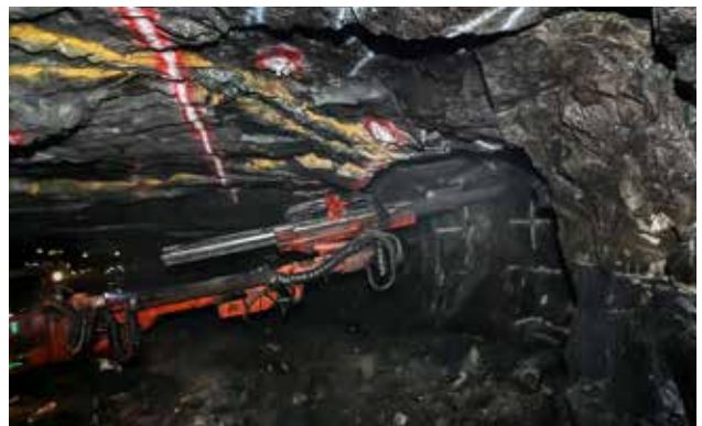
Drill and Blast Excavation
