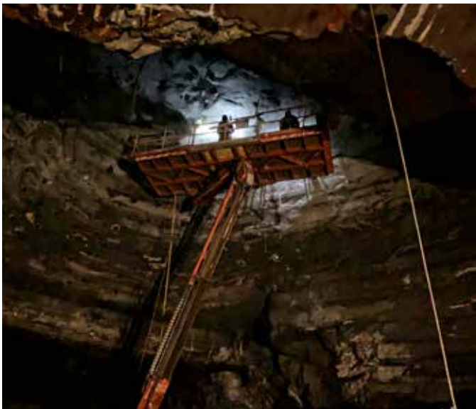
Installing 50 ft Cable Bolts
