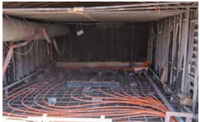
Track installed with heat tubes
