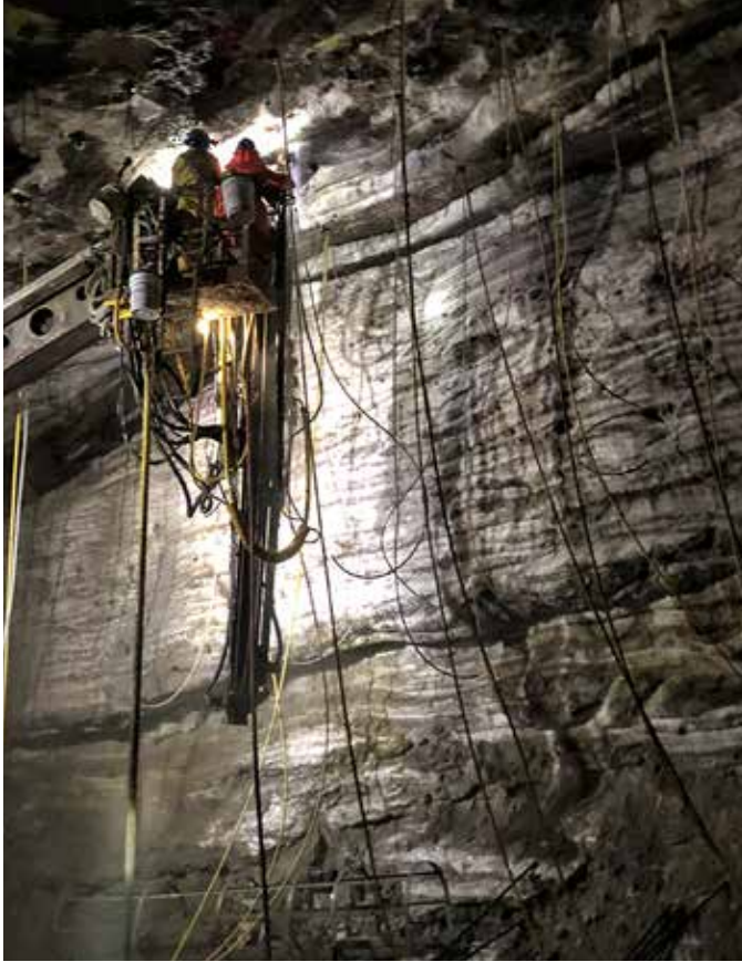
Installing 50 ft Cable Bolts
