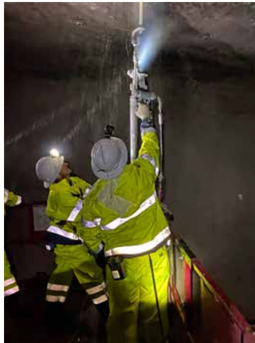
Installing 8 ft Point Anchor Bolts
