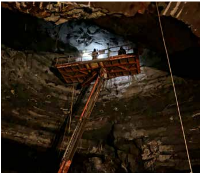
Installing 15m Cable Bolts
