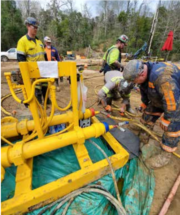
After Grout: The grout sealed up the pathways eliminating any further water ingress.
