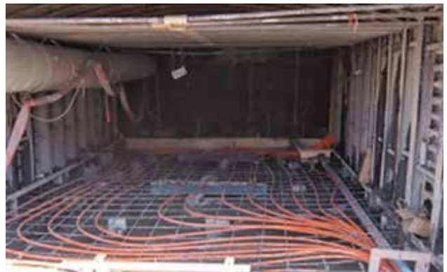
Track installed with heat tubes
