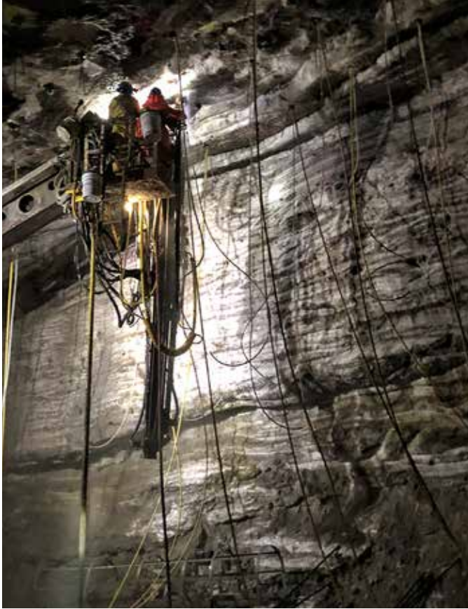
Installing 15m Cable Bolts
