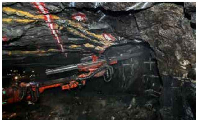
Drill and Blast Excavation
