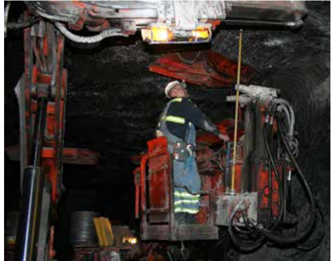
Installing 8 ft Point Anchor Bolts
