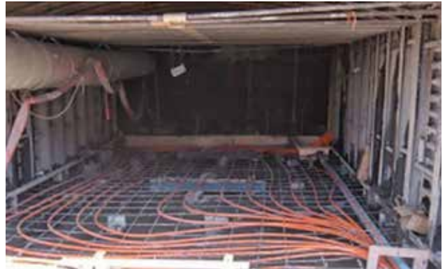
Track installed with heat tubes
