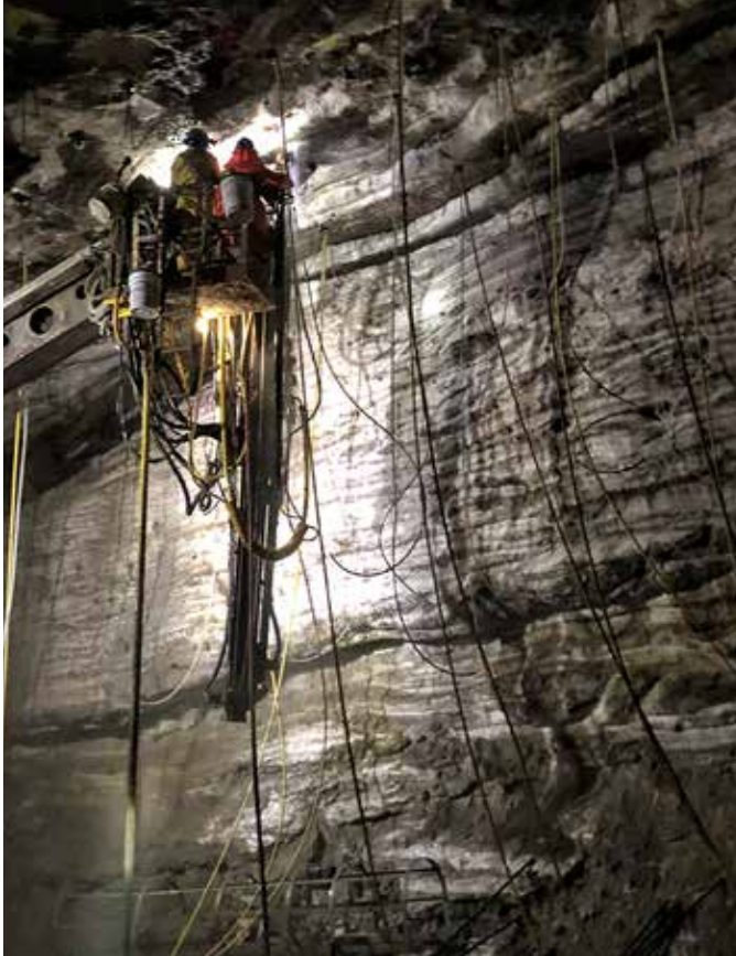
Installing 50 ft Cable Bolts
