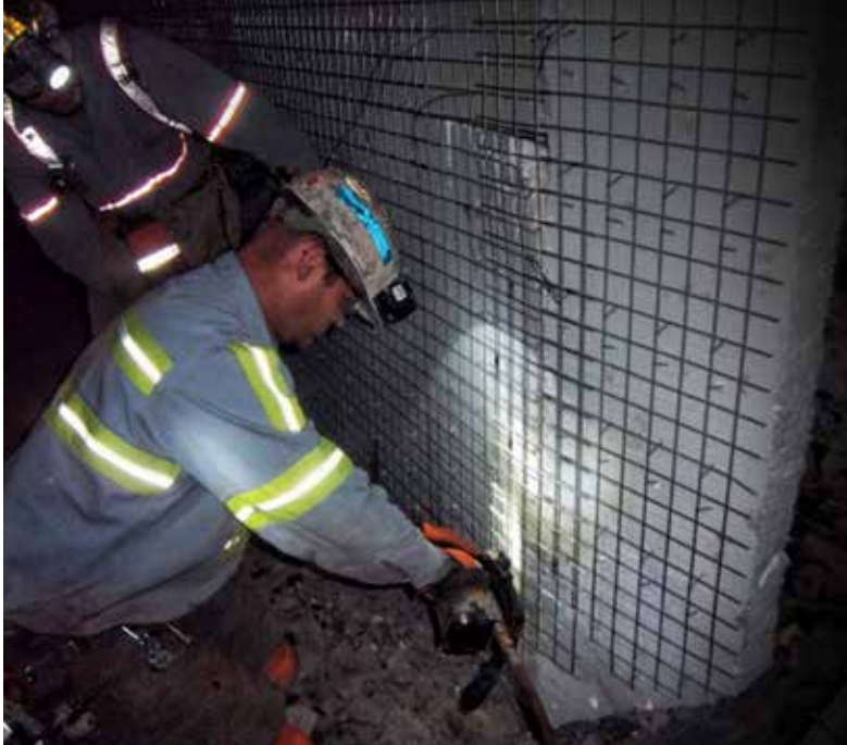
Sprayed Shotcrete high-pressure stoppings can withstand 22 in. wg
