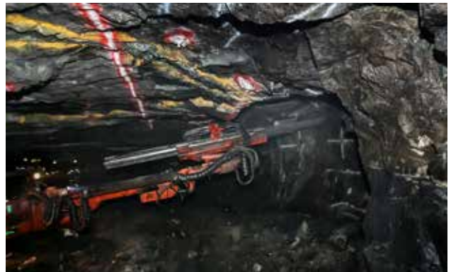
Drill and Blast Excavation
