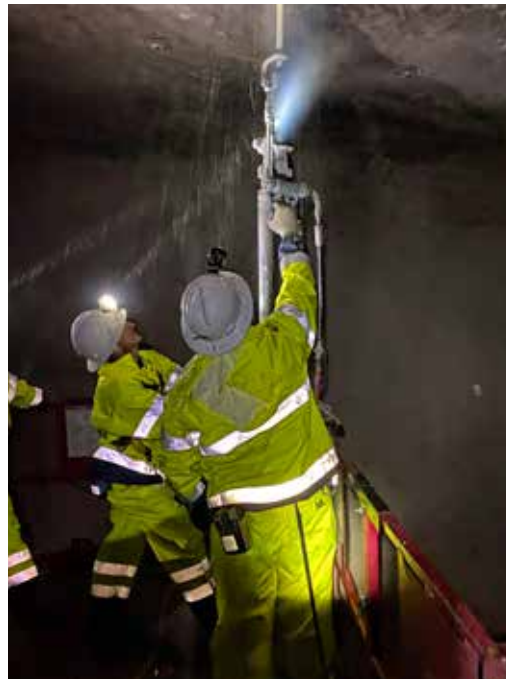
Installing 8 ft Point Anchor Bolts
